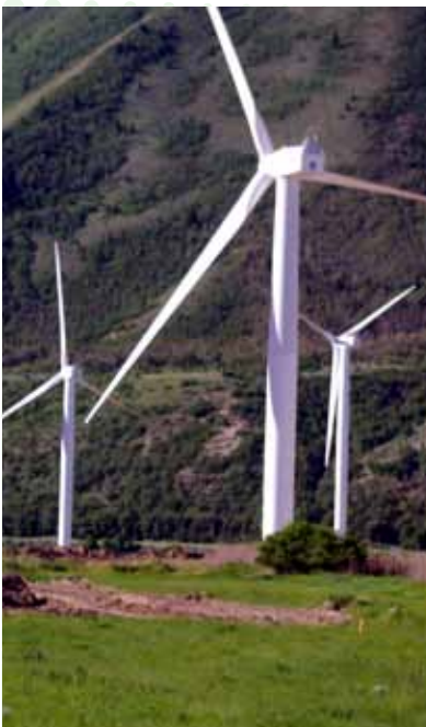
Edison Mission Energy Spanish Fork Windfarm - Utah Image used with permission of Edison Mission Energy
