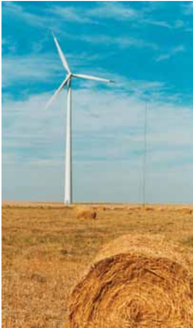
Xcel Energy Peetz Windfarm - Colorado Image used with permission of Xcel Energy
