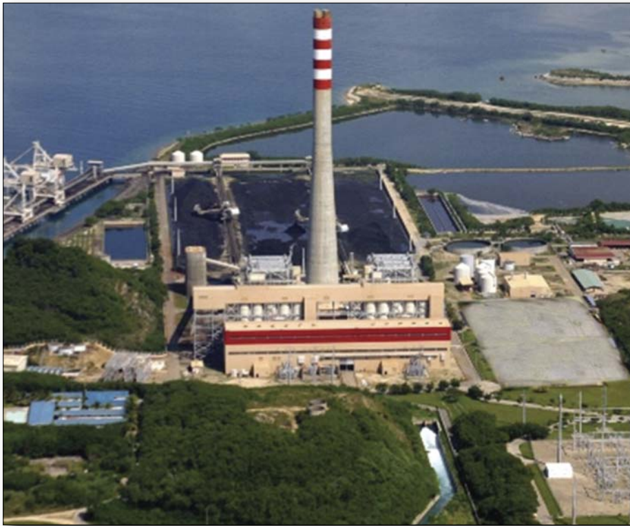
Figure 2: The Pagbilao coal plant in the Philippines operates with steam turbines by Mitsubishi Hitachi Power Systems
