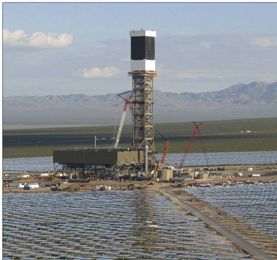
Figure 4: Ivanpah solar plant in California
