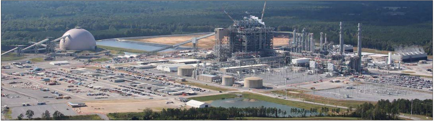
Figure 1: Mississippi Power's Kemper County Energy Facility
