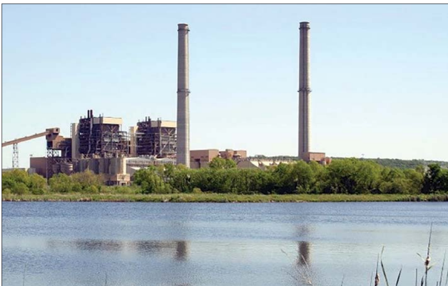
Figure 2: The Grand River Dam Authority facility in Oklahoma
