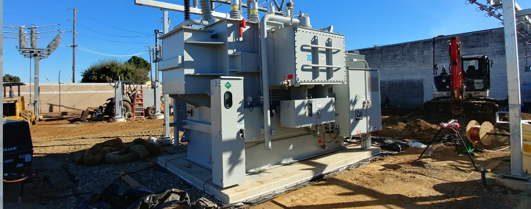
This new transformer at the Oregon Street Substation will receive power at 115 kilovolts (kV) and step it down to 12 kV for distribution to local homes and businesses.
