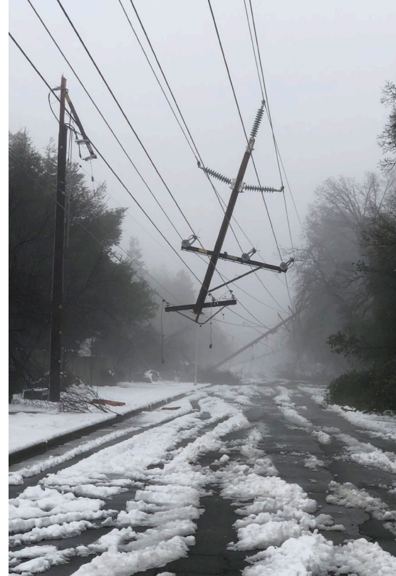
The February 12th storm snapped 14 transmission poles in REU's service area.
