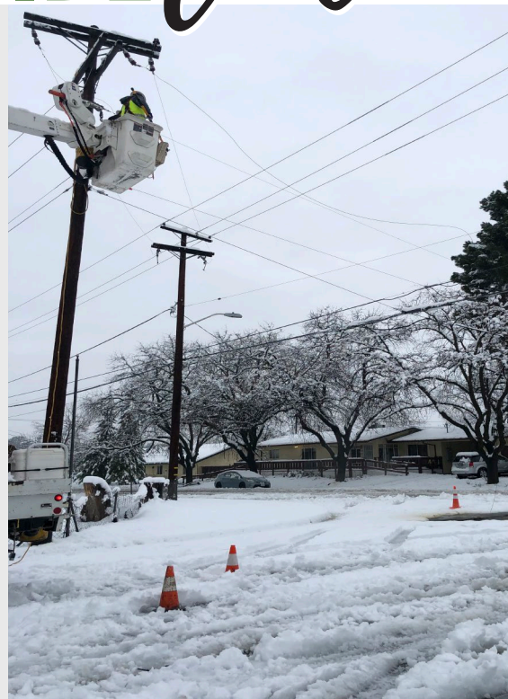
REU Linemen Dustin Hamilton and Jake Pearson work in a bucket truck to reattach a line following the February 12th snowstorm.
