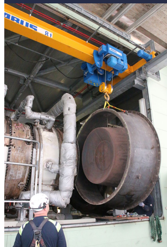
Contractors from Siemens dismantling and hoisting sections of the Unit 5 turbine.
