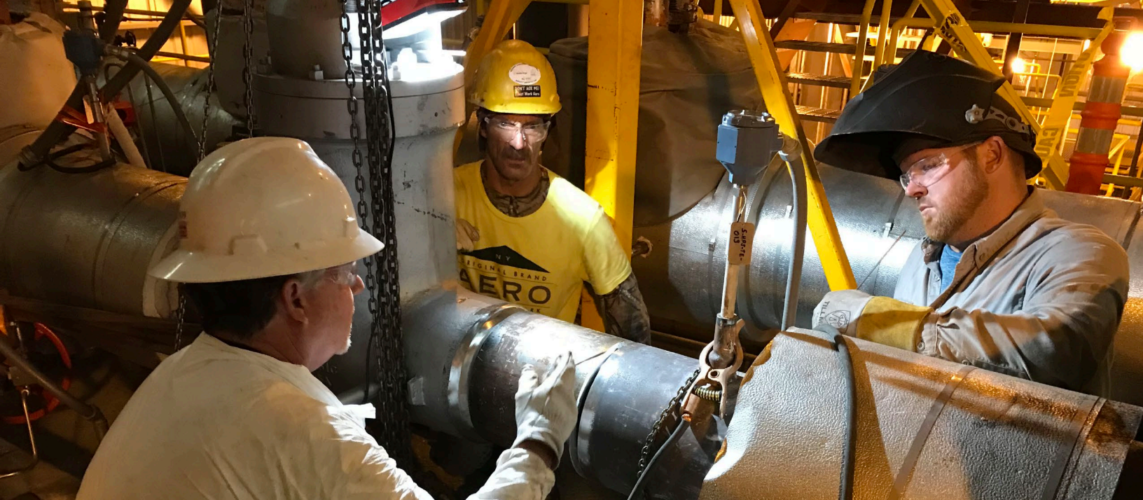
Redding Power Plant contractors aligning the new Unit 4 steam turbine valve.
