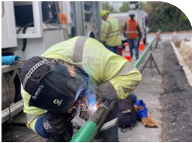
A CPAU Utility worker replacing a natural gas main.
