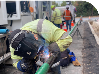
A CPAU employee replacing a natural gas main.
