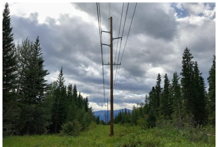
Figure 4: 69-kV covered conductor is available in tree wire or spacer cable configurations
