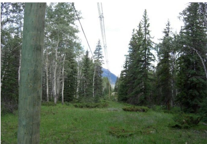
Figure 3: To comply with narrow rights of way imposed by Canada's Jasper National Forest, ATCO Electric used Hendrix distribution and transmission lines.—Source: ATCO
