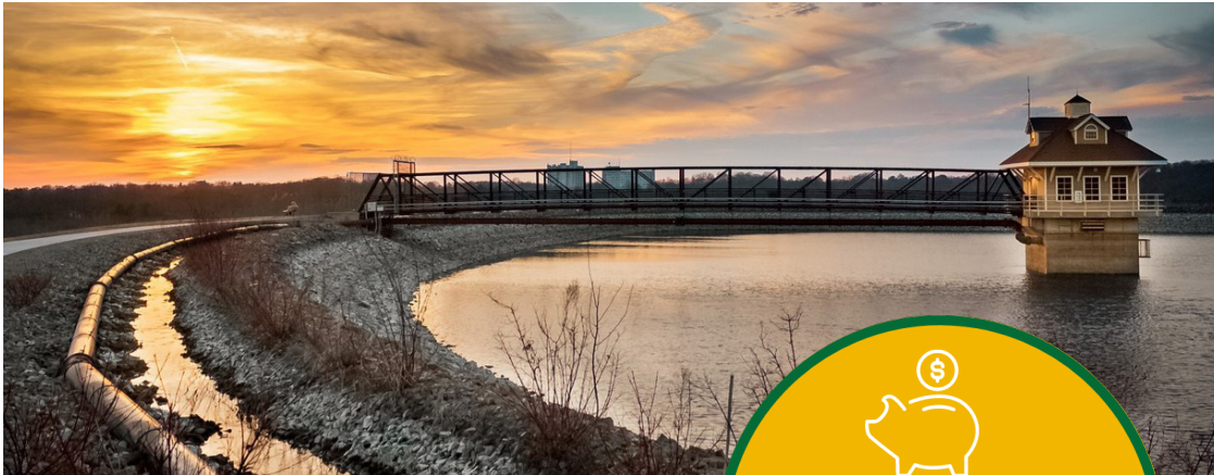
Newark Reservoir, Newark, Delaware
